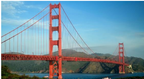
Golden Gate Bridge
